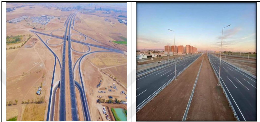
Figure 3.5: Highway No. 3 (150-Meter Erbil)
