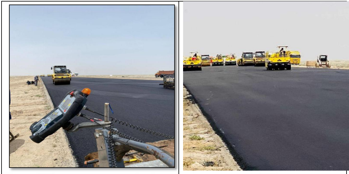
Figure 3.3: Highway No.1 Samawah- Nasiriyah Road
