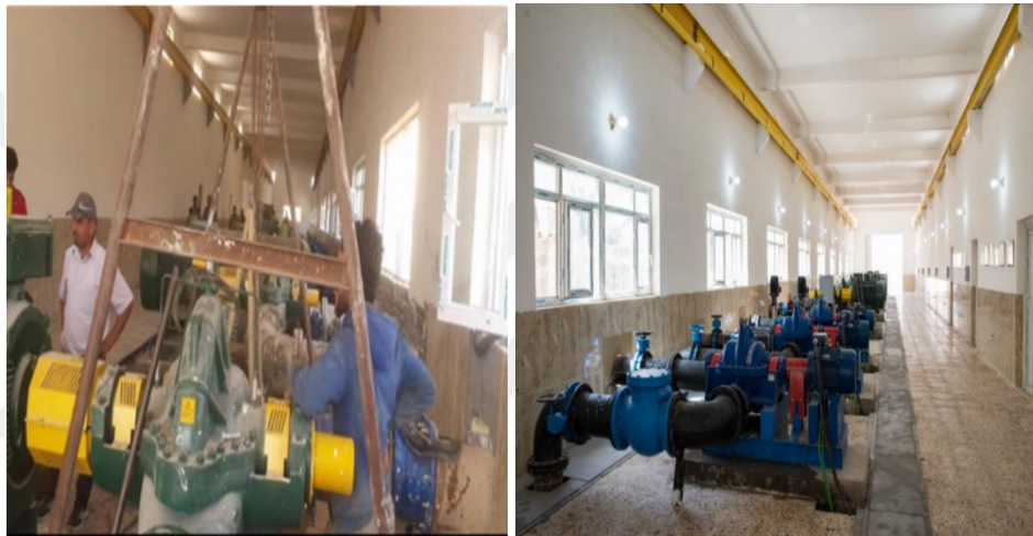
Figure 3.2: AL-Azrakiyah DWTP after Rehabilitation in 2017
