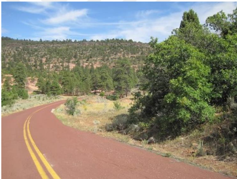
Figure 4.28: Red Coated Asphalt
