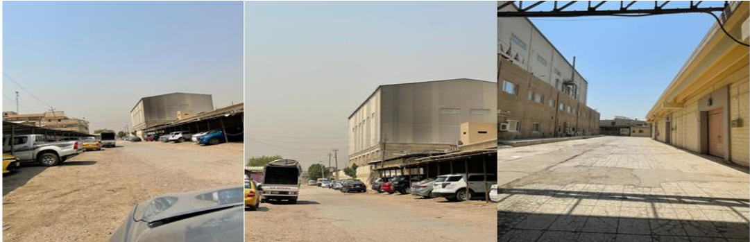
Figure 4.7: Selected Building (Printing House Al Sabah Newspaper )
