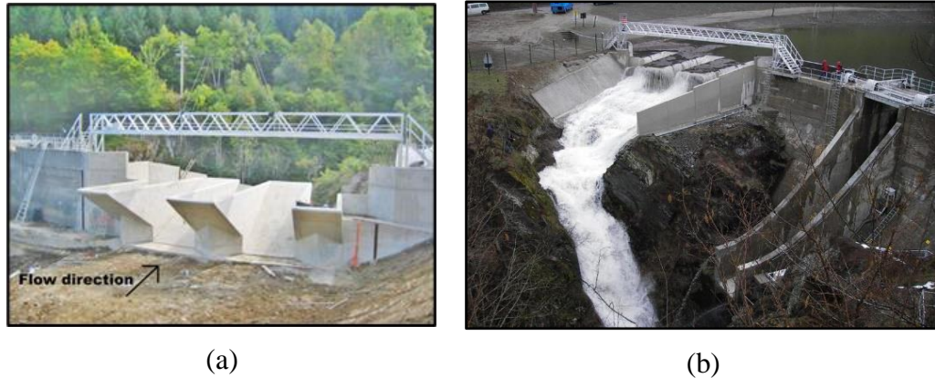
Figure 1.4: The PKW system at the EDF Goulours dam in France.
