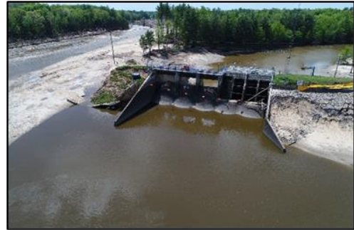
(b) The Edenville Dam Failure in Michigan, USA.
