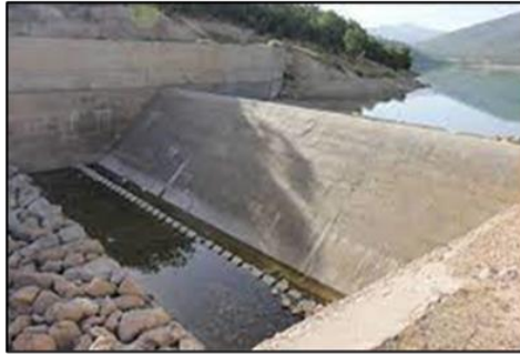
(a) Ogee weir (Shahghasem dam in Iran).
