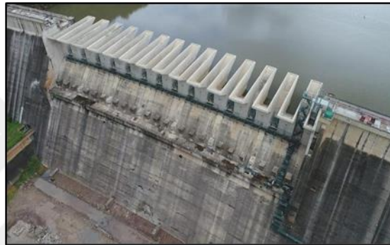
(c) Piano Key Weir (the Hazelmere Dam in South Africa).
