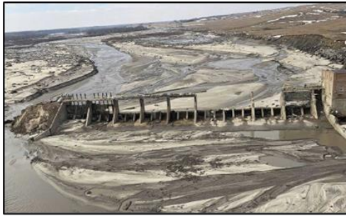
(a) The Spencer Dam Failure in Nebraska, USA.
