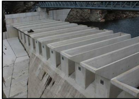
Figure 1.3: Malarce Dam in France
