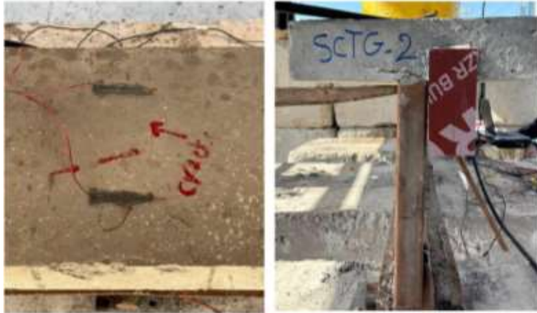
Figure 6.9: Crack Pattern of the SCTG-2
