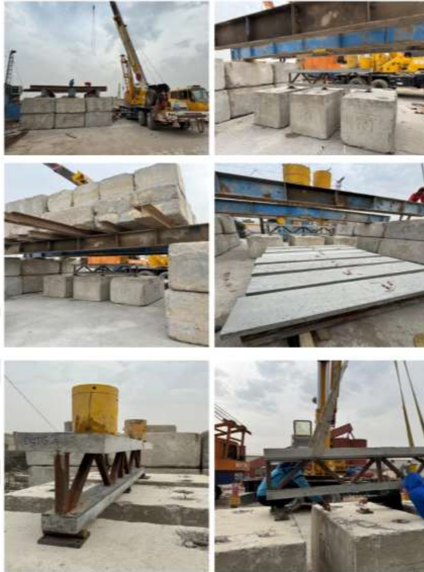
Figure 4.45: Hydraulic Jack and Load System Installation
