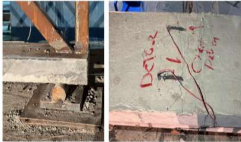
Figure 6.33: Initial and Ultimate Cracks Pattern of the DCTG-2
