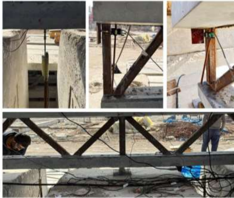
Figure 4.42: Site Installation of the LVDT Indicator for Category Two Specimens (DCTG)
