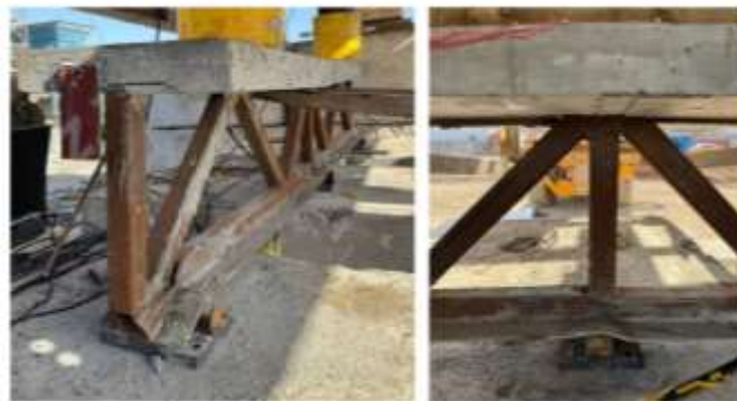
Figure 6.4: Failure Mode of the SCTG-1
