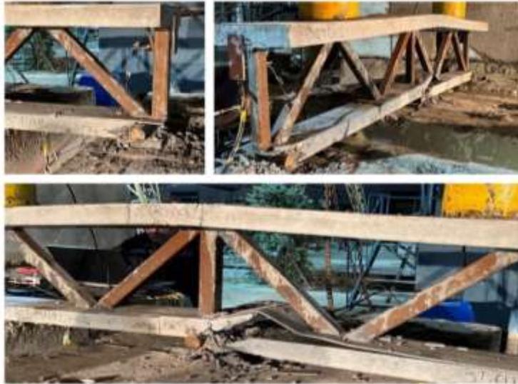
Figure 6.28: Failure Mode of the DCTG-1
