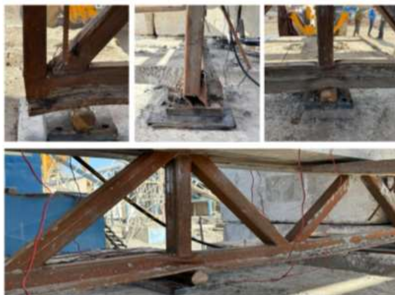
Figure 6.5: Failure Mode of the SCTG-2
