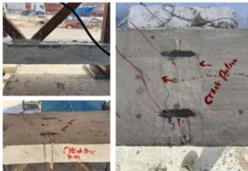
Figure 6.35: Initial and Ultimate Cracks Pattern of the DCTG-4
