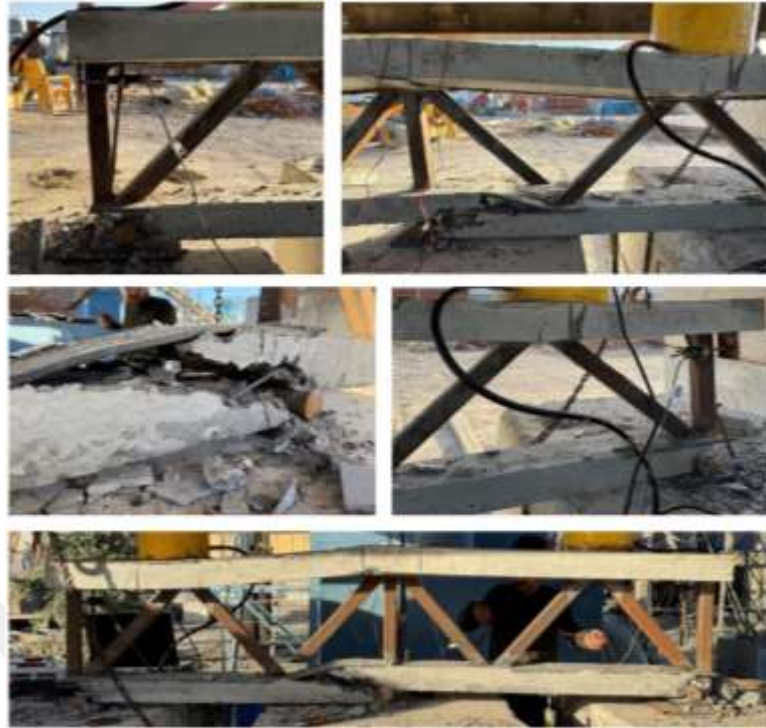
Figure 6.30: Failure Mode of the DCTG-3
