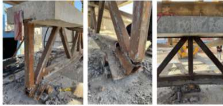
Figure 6.6: Failure Mode of the SCTG-3
