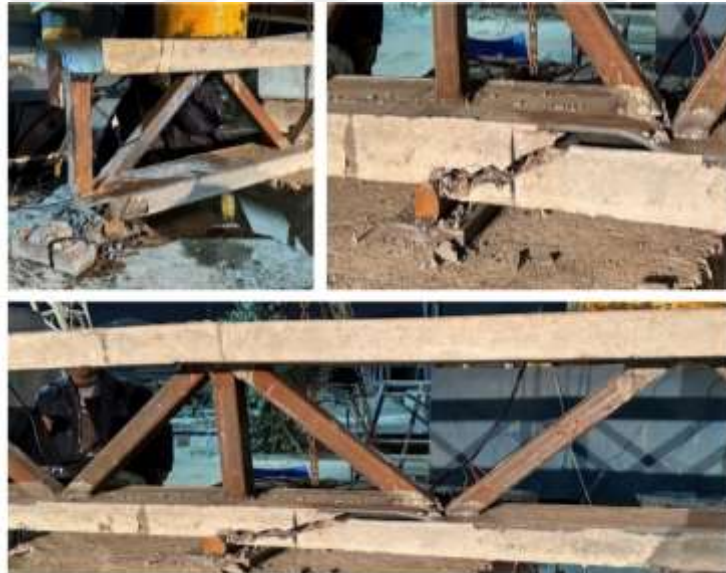
Figure 6.29: Failure Mode of the DCTG-2
