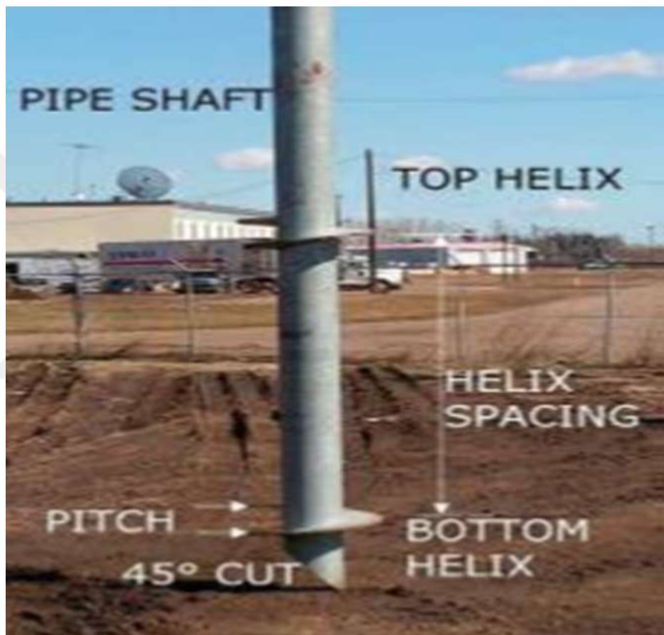
Figure 1.1: A Screw Pile Geometry
