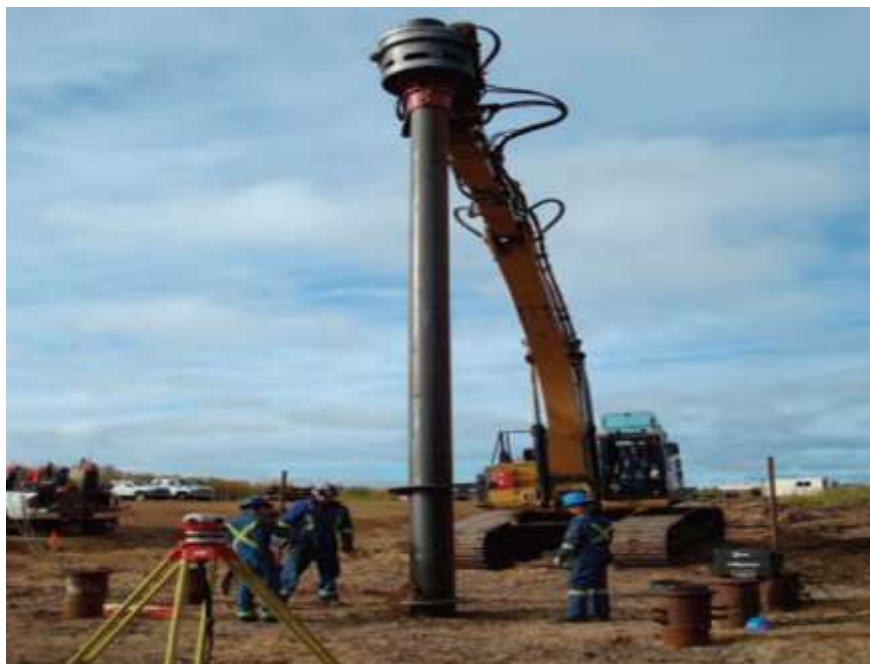
Figure 2.2: Helical Pile Placement Field Apparatus [45]
