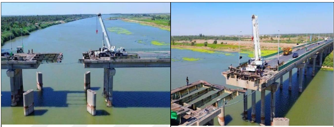
Figure 3.2: Numaniyah Concrete Bridge in Wasit (RW)
