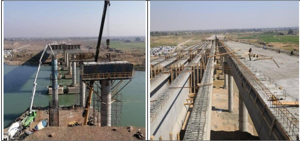
Figure 3.9: North Tikrit Bridge (Study Sample) (RW)
