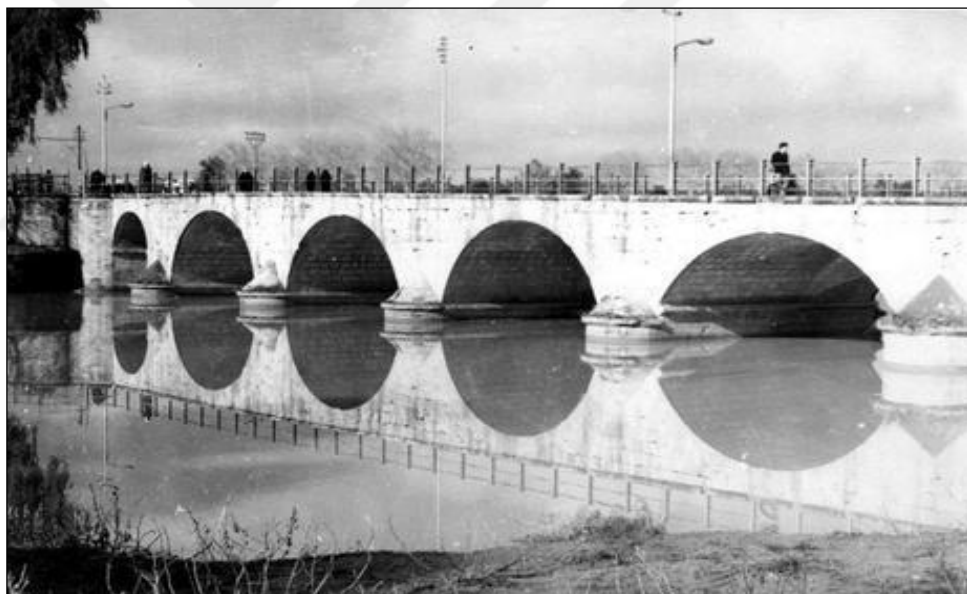
Figure 2.2: Stone Arch Bridge
