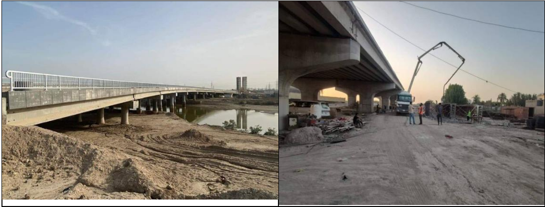
Figure 3.1: North Nasiriyah Bridge in Dhi Qar (RW)
