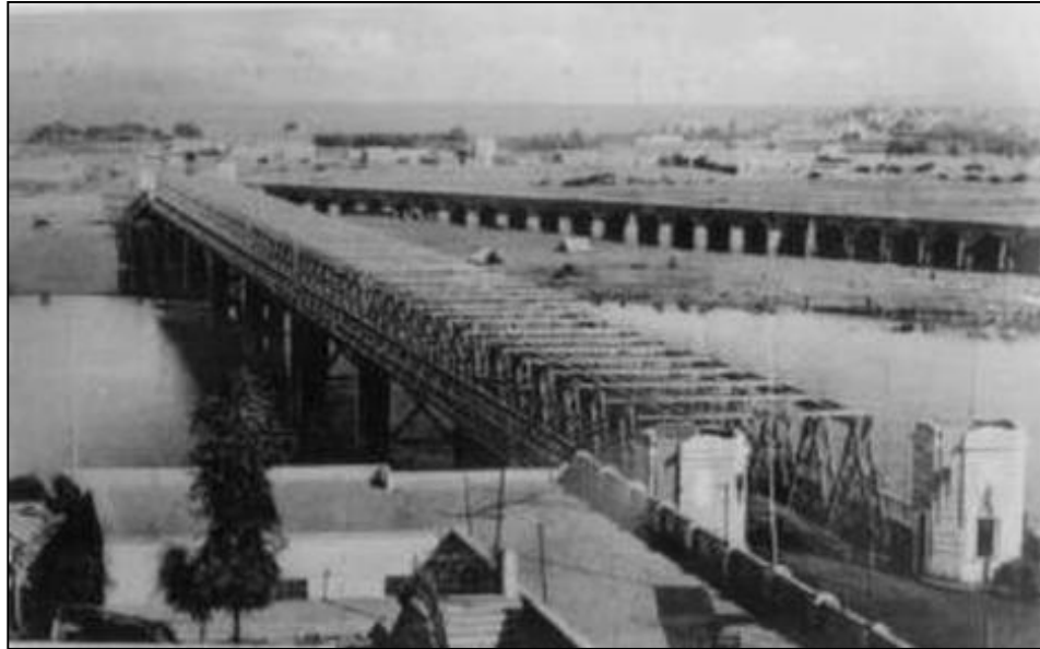
Figure 2.1: The Old Bridge (Antique)
