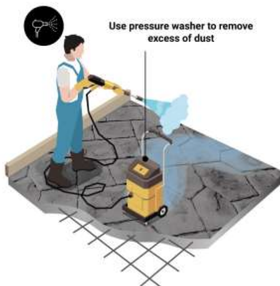
Figure 3.12: The Stamped Floor Screed
