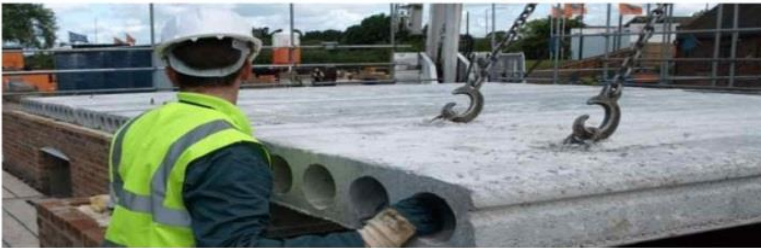
HOLLOWCORE BEING ERECTED / INSTALLED
