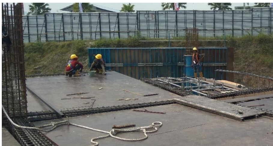
Figure 4.4: Slab and Beam Formwork Installation
