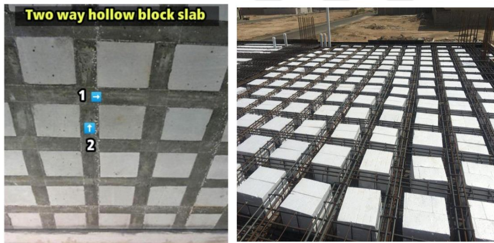
Figure 2.18: Site Implementation for Two-Way Ribbed Slab.
