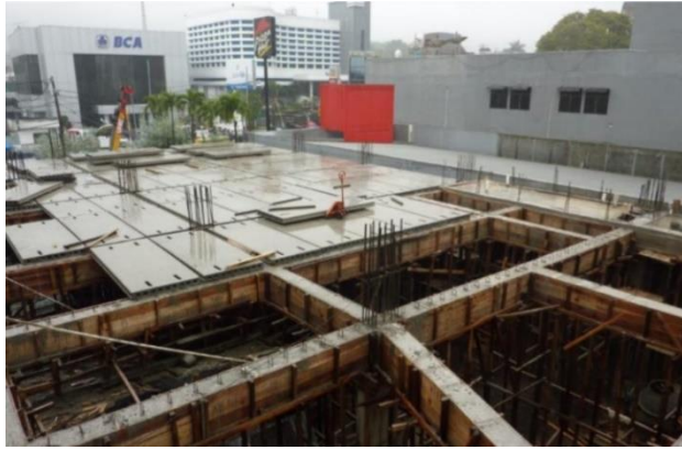
Figure 4.12: Precast Hollow Core Slab Panels Installation Works
