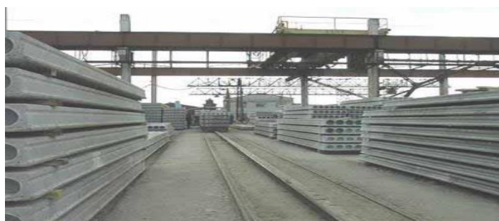
Figure 2.29: Storage in the Precast Production Plant
