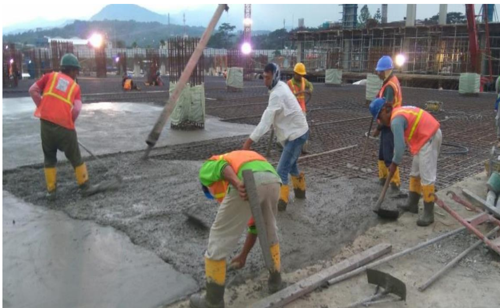
Figure 4.6: Casting of Slabs and Beams with a Concrete Pump
