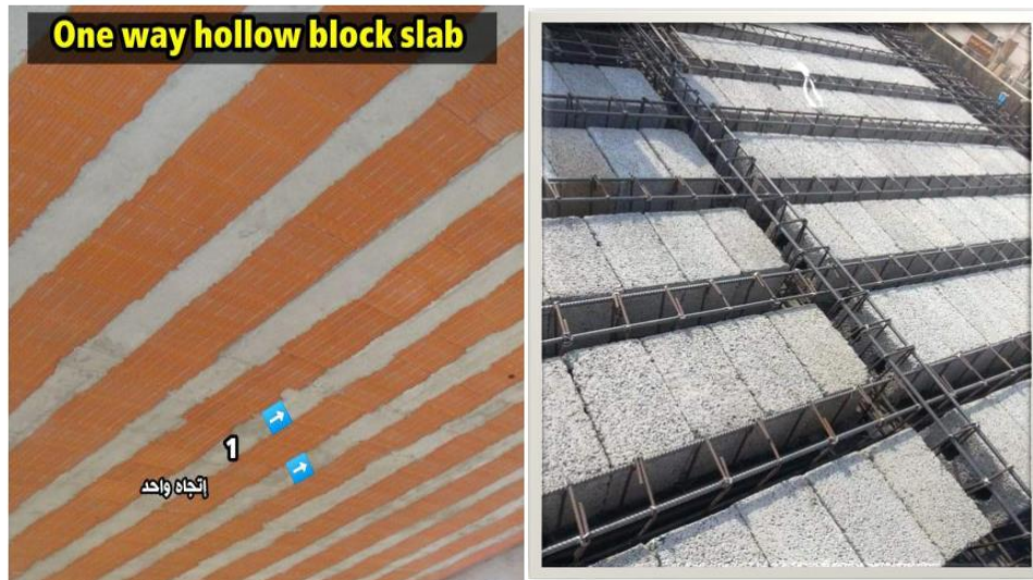
Figure 2.14: Site Implementation for One-Way Ribbed Slab
