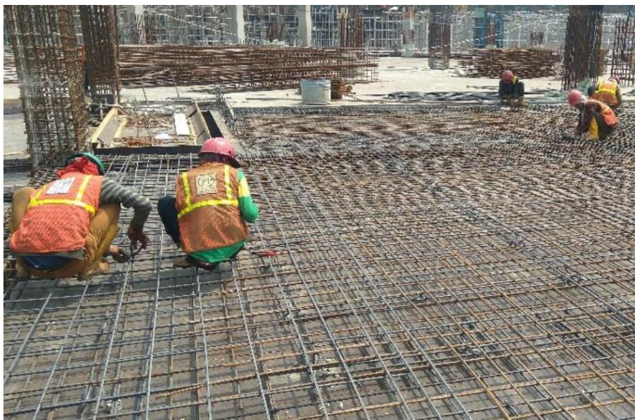
Figure 4.5: Reinforcement of Slabs and Beams
