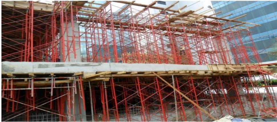
Figure 4.3: Scaffolding for Slabs and Beams
