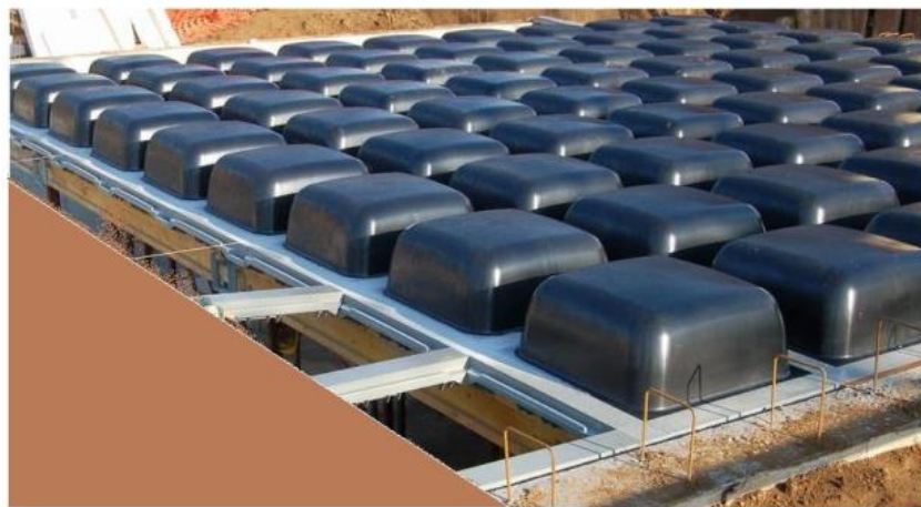
Figure 2.16: Waffle Slab Formed Using Steel Pans
