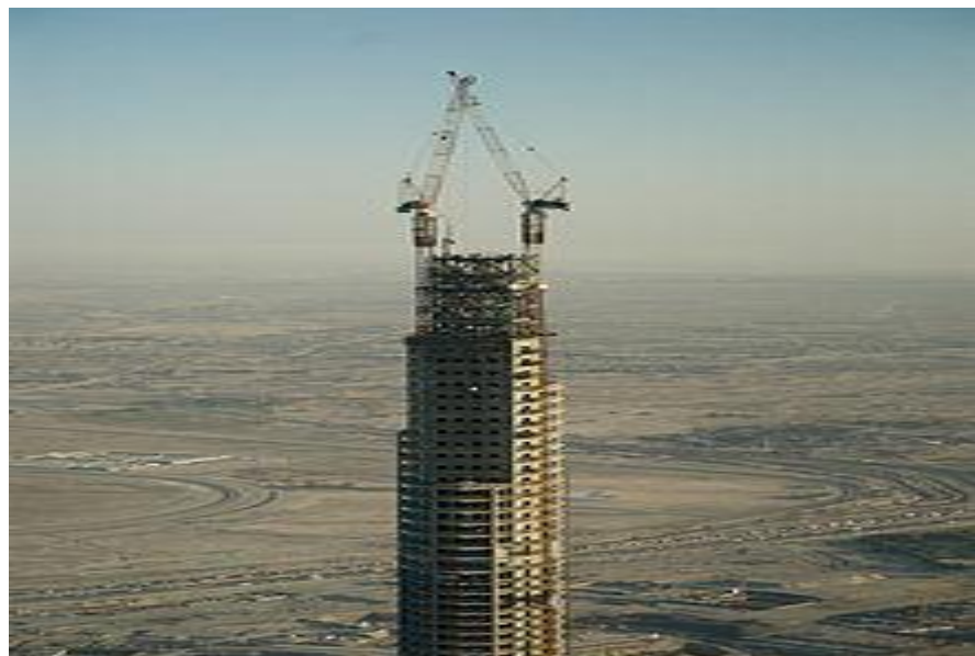
Figure 2.2: Burg Khalifa, the World's Tallest Building
