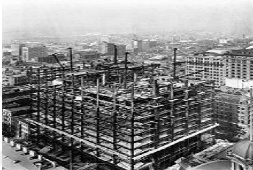
Figure 2.1: Woolworth Building Under Construction in 1912
