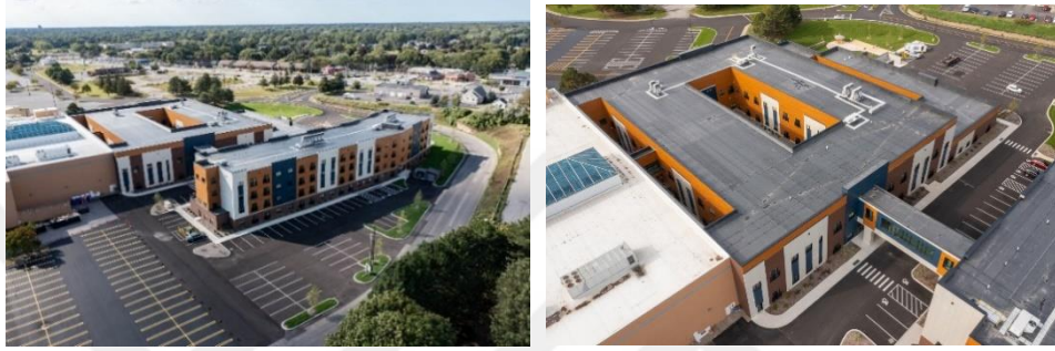
Şekil 4.50: Skyview Park Apartments
