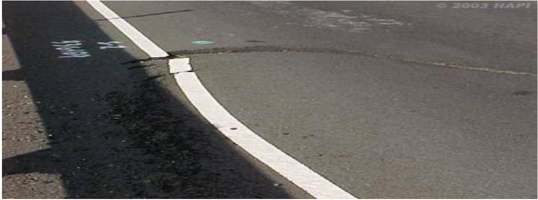
Figure 2.6: Slippage Cracks
