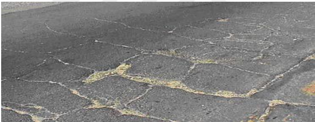
Figure 2.3: Block Cracks
