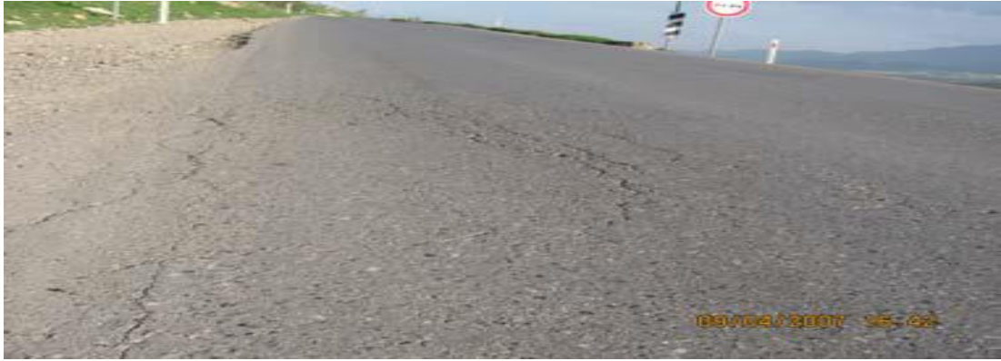
Figure 2.4: Edge Cracks
