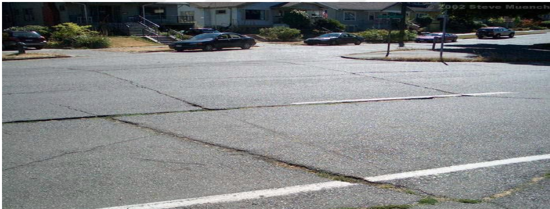
Figure 2.5: Reflection Cracks
