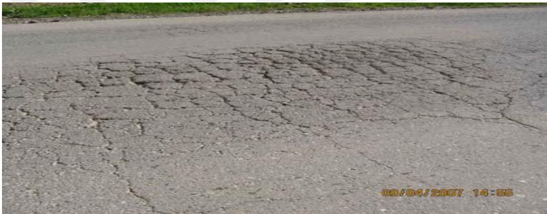
Figure 2.1: Alligator Cracks
