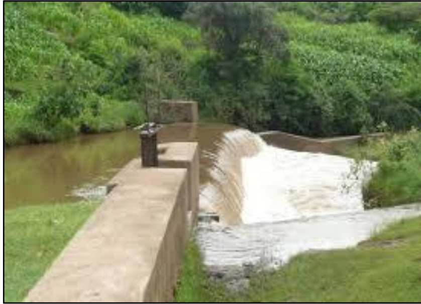
Figure 4.2: The Floodwater Harvesting System
