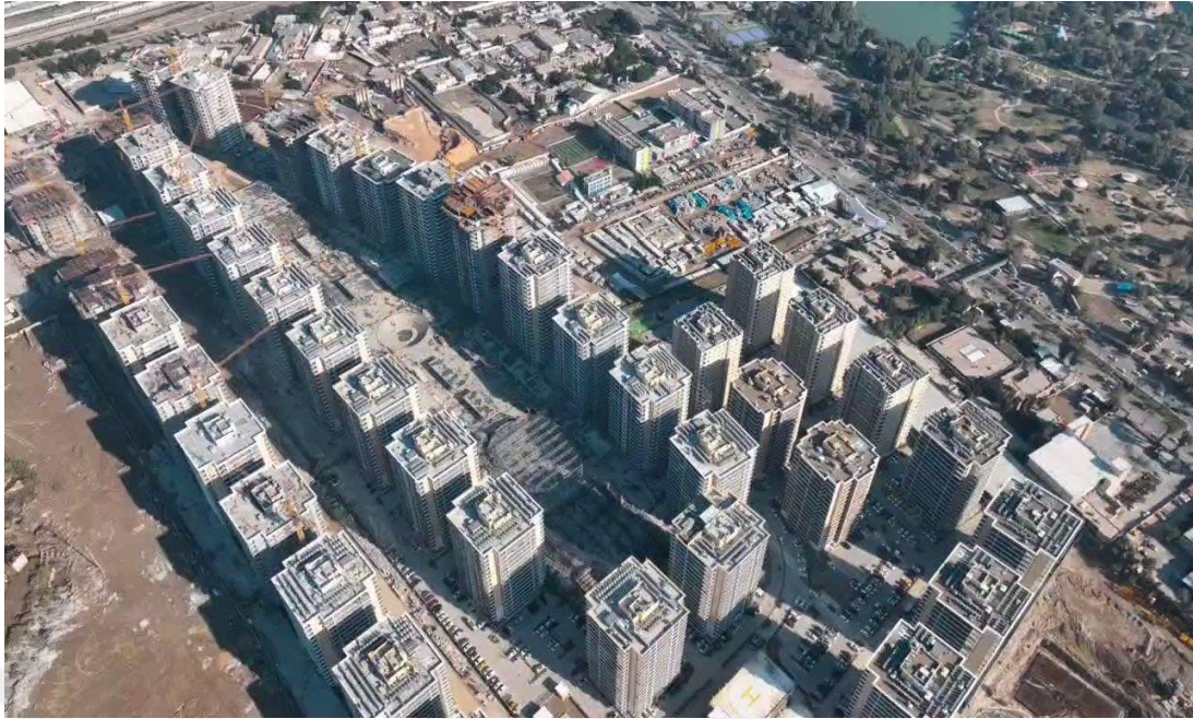
Figure 4.6: Iraq Gate Residential Complex
