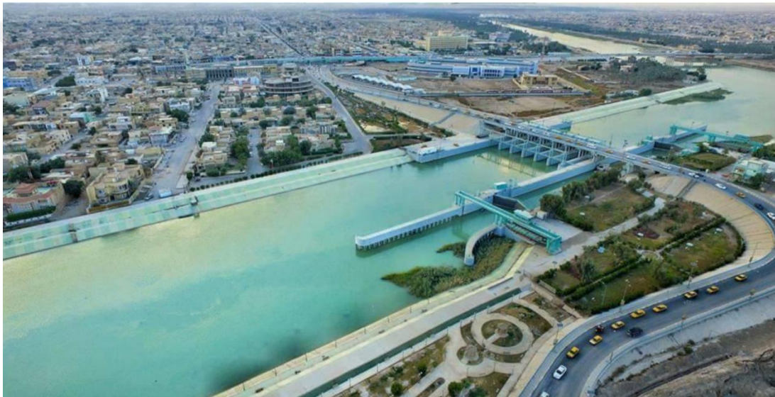
Figure 2.6: General view of Amarah Barrage
