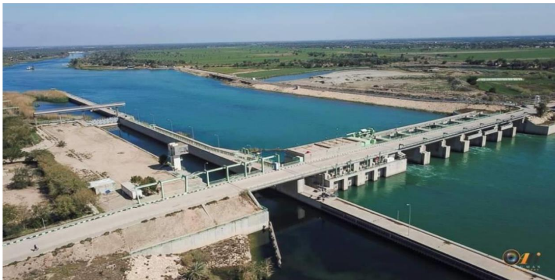
Figure 2.8: General view of Kufa Barrage
