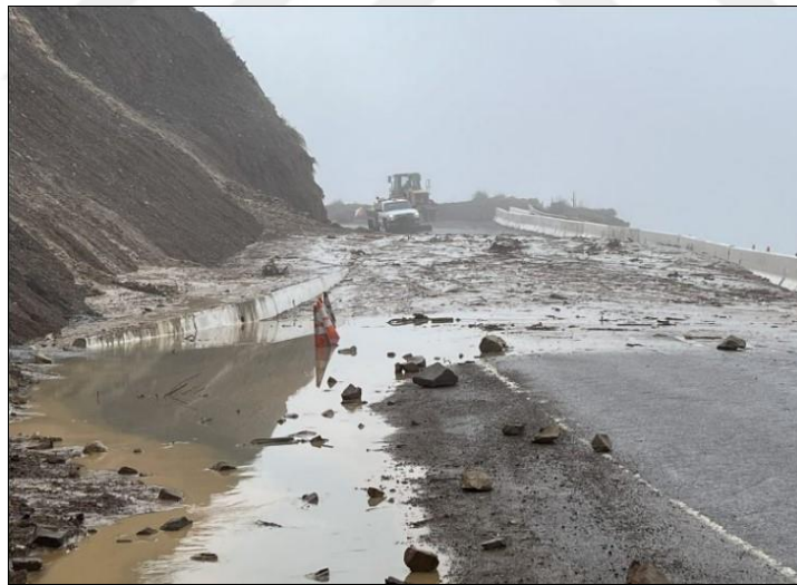
Figure 2.9: Damage to Highway 1 in Monterey County, California, March 2023
