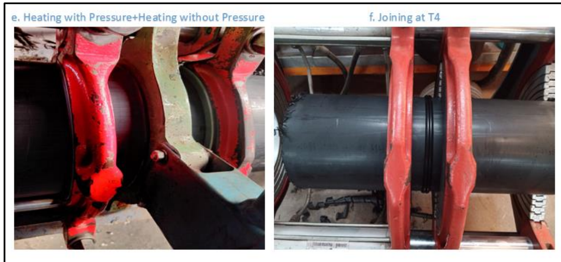
Figure 6.11: Heating (e) and butt fusion (f) of pipe samples
