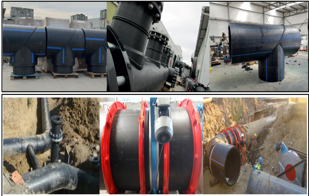
Figure 2.2: HDPE pipe installation and butt fusion welding
