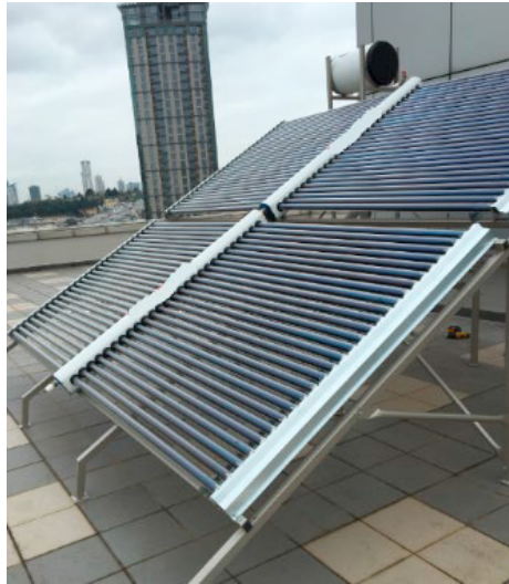
Figure 1. The evacuated tube heat pipe collector
