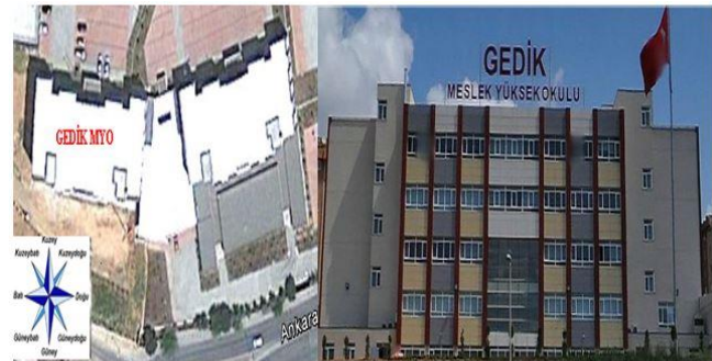
Fig.2. Satellite and front view of the IGUVS building.
