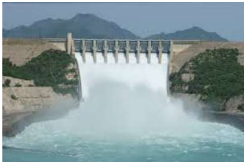
Figure 4.13: Kurram Tangi Dam Project Spillway
