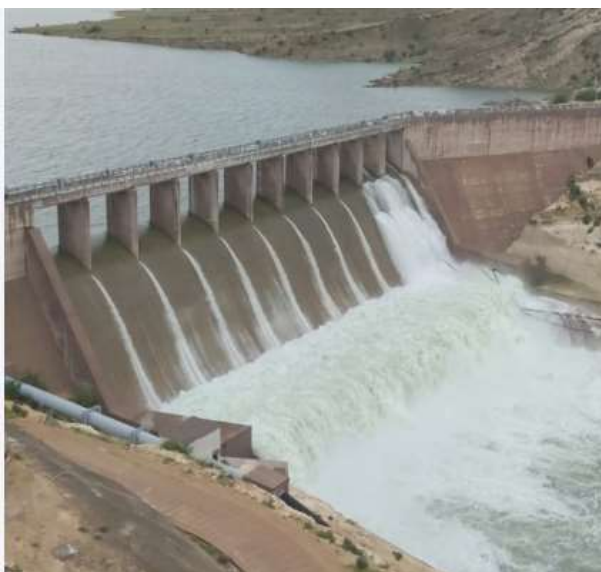
Figure 4.8: Darawat Dam Spillway
