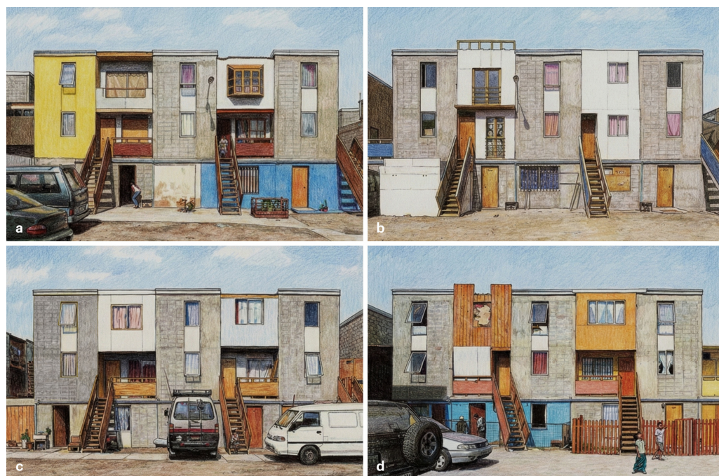
Figure 8. Unique facade variations generated by users according to their socioeconomic means and aesthetic preferences. (a) [28]; (b) [29]; (c) [30]; (d) [31]. (Redrawn by the authors based on [28–31]).
